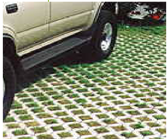
Pervious surface is ideal for overflow parking Center for Watershed Protection
